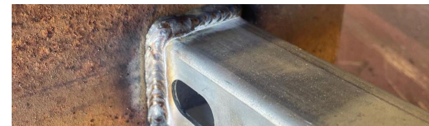
Welding galvanized steel to rusty steel using Tartan B MIG
