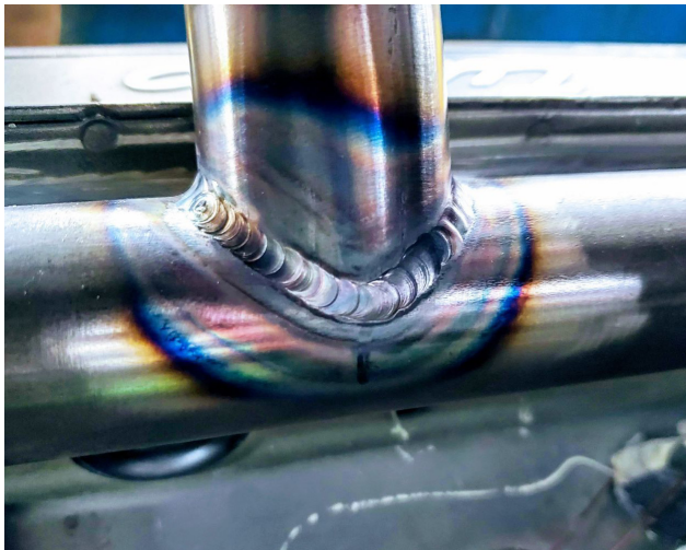
Brutus TIG used here to construct a chromoly steel roll cage. Brutus can weld any steel.
